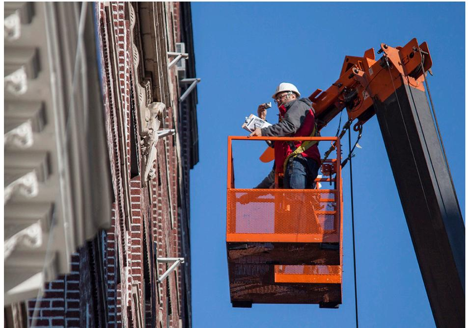
But there are alternatives that can be both cheaper and more effective than scaffold drops. One alternative is rappellers who use ropes to drop from roof to ground, inspecting the facade as they descend. Another is bucket trucks, also known as “boom trucks” or “boom lifts,” and commonly used by firefighters.
